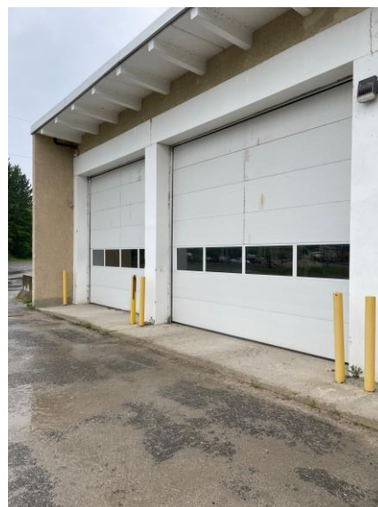
Photo 3. Bathurst Garage, Insulated Doors
