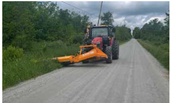
Roadside grass is cut back from the shoulder in June and July to provide proper driving sight lines
