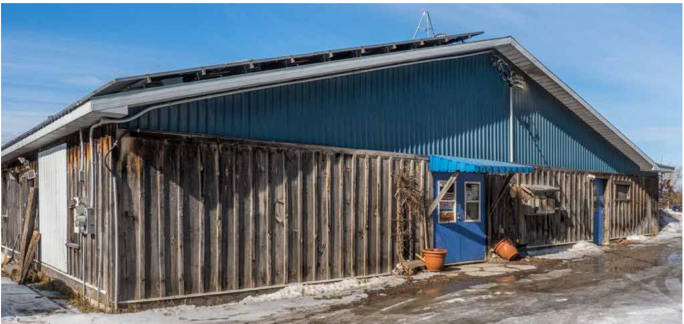
Figure 1 South side view of the Chaplin Dairy
